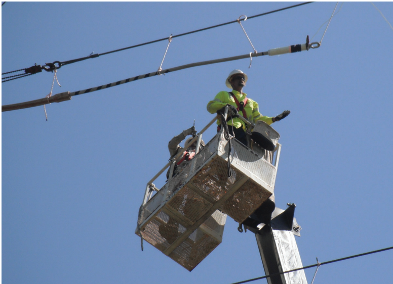
Workers prepare an implosive connector for detonation.
