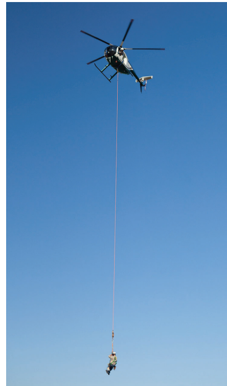
A utility lineman prepares to attach a spacer between transmission conductor.
