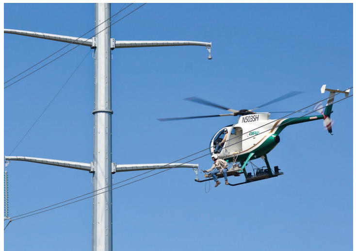
Above. A utility lineman attaches a spacer between transmission conductor.
