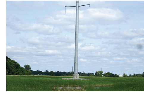
Native vegetation in the Bel Claire Marsh near St. Cloud is reestablishing less than six months after a structure was constructed for the Monticello-St. Cloud project.
