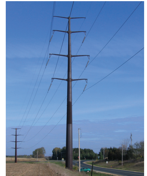
Structures similar to the tower pictured here will be spaced between 800 and 1,000 feet apart.
